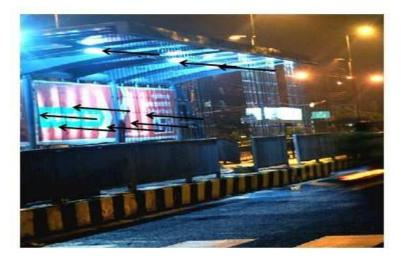
Figure 1: The 40 Watt T-12 Tube Lights on BRTS Stop, Indicated by Arrows
